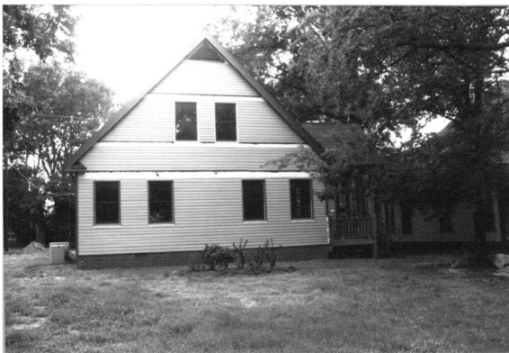
Figure 9: 1304 Cumberland St., east elevation, photo courtesy of Arkansas Architectural Resources Form, 1998.
