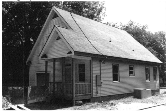
Figure 10: 1304 Cumberland St., southwest elevation, photo courtesy of Arkansas Architectural Resources Form, 1998.
